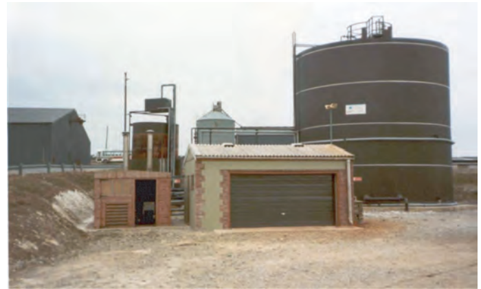
Figure 15.9 | Anaerobic digestion plant and biogas storage tank on a 4000-sow pig farming in South England using two gas engines (housed in the closed shed) to provide electricity for the farm as well as low-grade heat for drying Lucerne horse feed as an ancillary farm operation. Source: courtesy of Ralph Sims.
