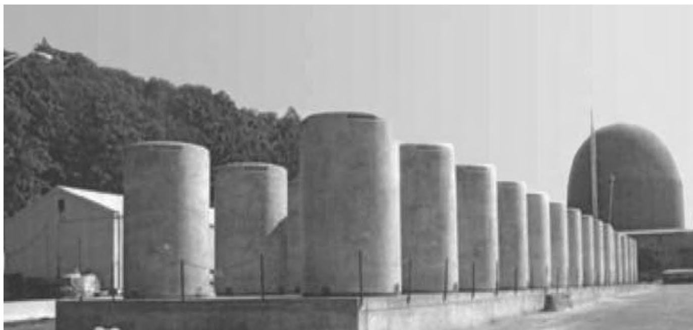
Figure 14.15 | Dry cask storage of older spent fuel at a US nuclear power plant. Each year, a 1000-MW e light-water reactor discharges spent fuel that originally contained about 20 tonne of uranium. Each cask typically holds about half that amount and costs US 2005 $1–2 million. Reprocessing spent fuel costs about ten times as much. Source: Connecticut Yankee, 2008.
