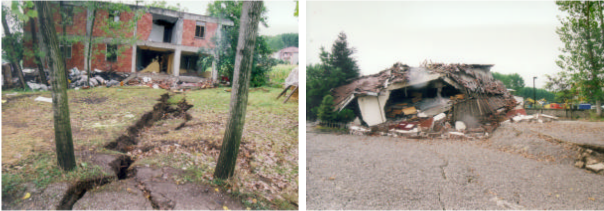
Figure 4. Collapsed buildings in Yuvacik (east of Gölcük) being located astride the surface rupture
