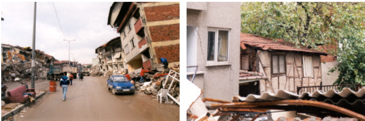
Figure 5. A scene within Adapazari city: a) damage of "engineered" RC-frame structures, b) traditional building type (timber framework) in the vicinity
