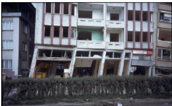
Figure 7 (left) Structural failure (soft storey) of a group of similar buildings
