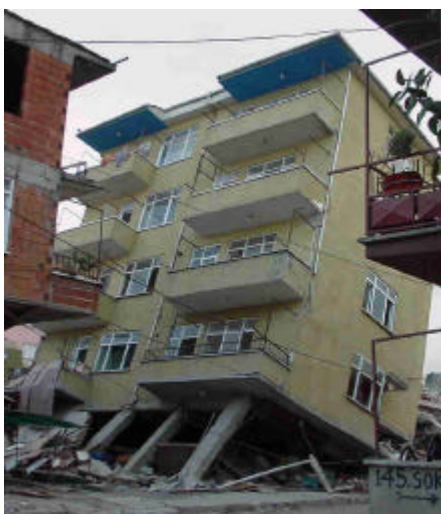
Figure 6 (right) Partial collapse of building due to failure of cantilevered floor slabs
