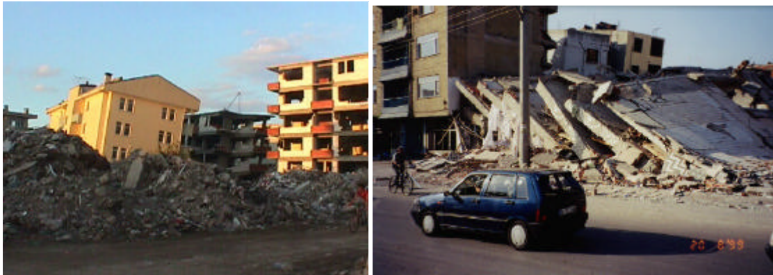
Figure 9 (left) Various levels of damage: from complete disintegration (rubble in foreground) to soft storey failures to collapse of external masonry walls
