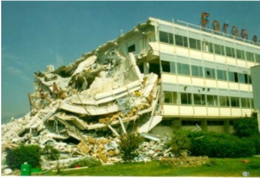
Photo 1. Partial collapse of an industrial complex (Faran SA).
