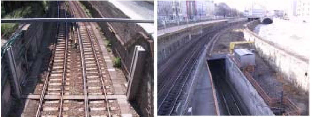
Figure 2: Portable Flood Barriers. Left: Naschmarkt; Right: Langenfeldgasse
